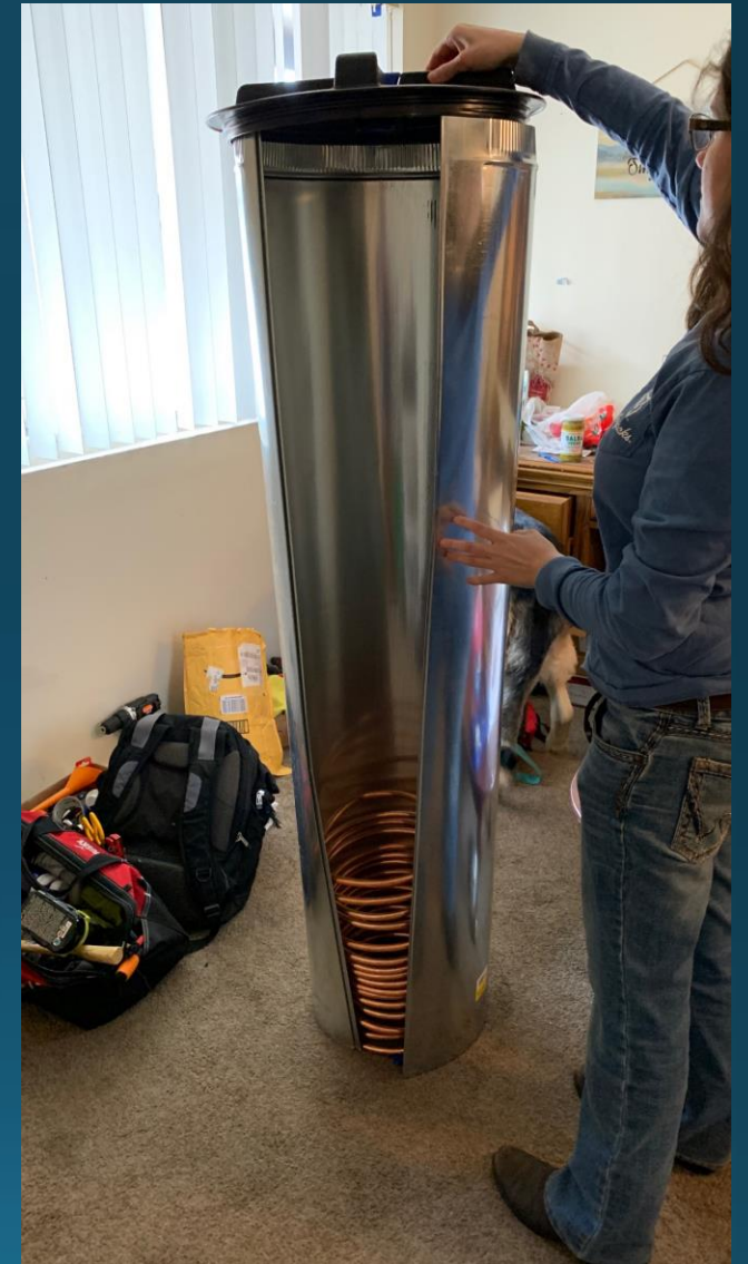
Figure 8: Ensuring that heat exchangers fit in the duct
